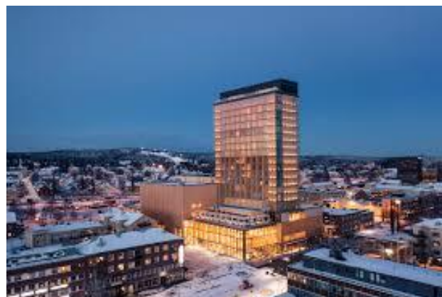
Figure 8: A High Rise Wood Framed Building Sweden
