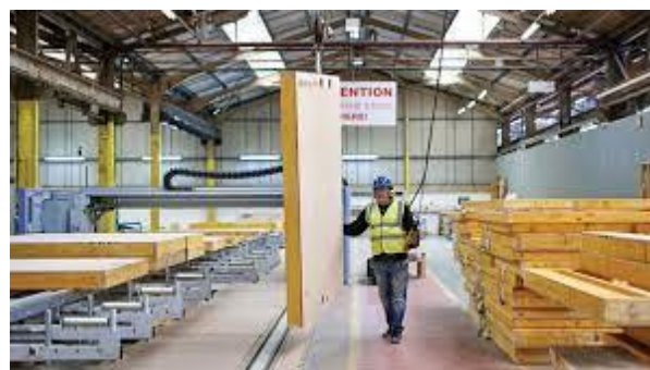
Figure 6: MMC Off-site Construction
