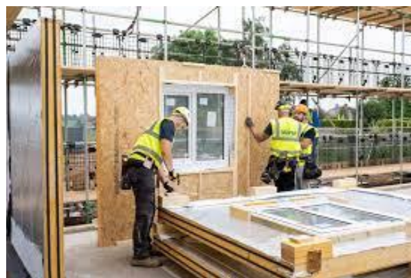
Figure 5: MMC assembling a wood framed house
